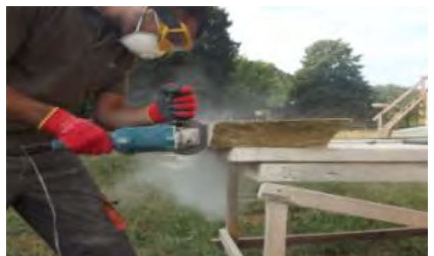
Fig. The stone cutting
