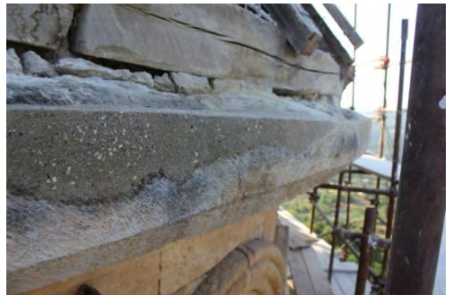
Fig. The cornice detail after the reconstruction
