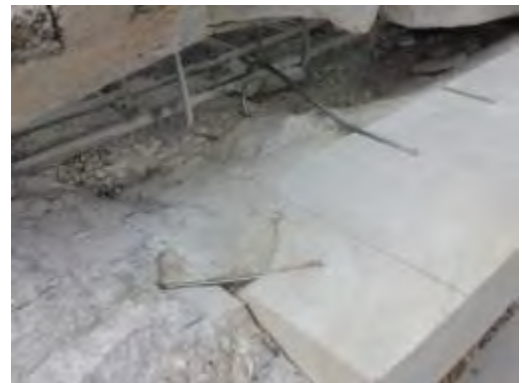
Fig. Anchored stone details
