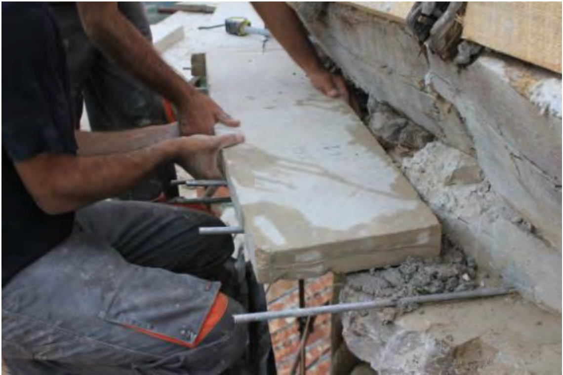
Fig. Fixing with the lime mortar
