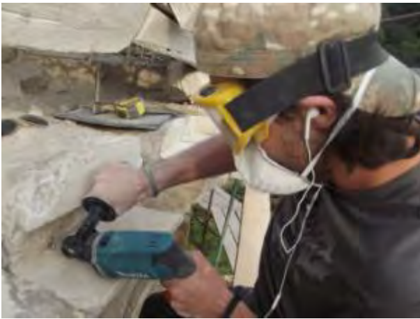
Fig. Preparing the holes for anchoring
