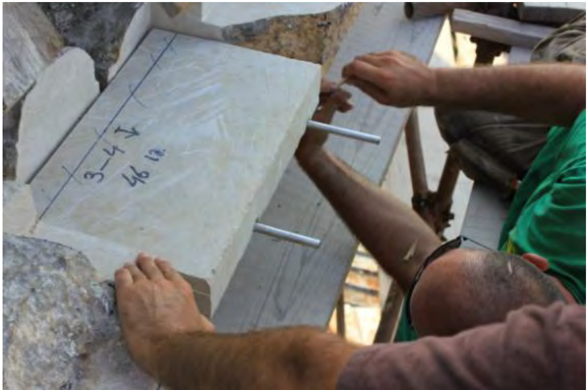
Fig. Fixing the stone
