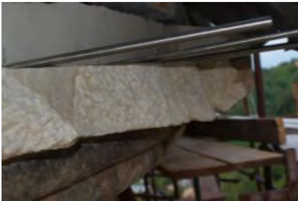
Fig. Treated stone surface
