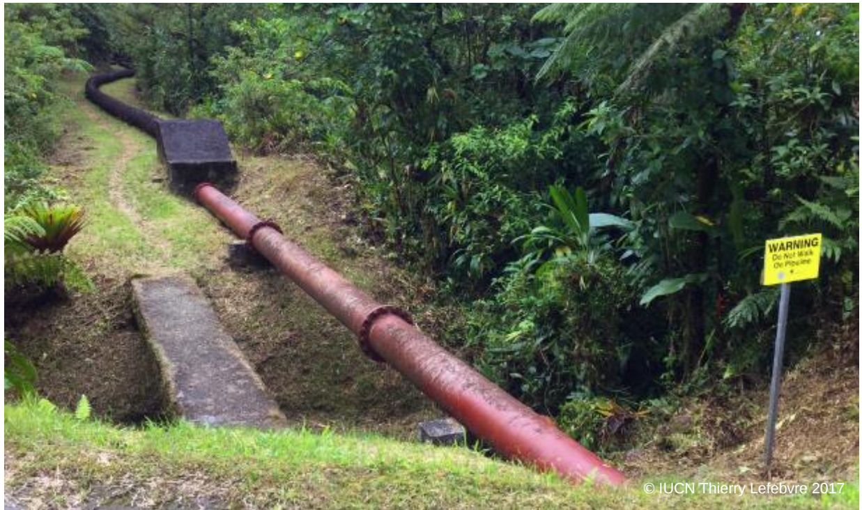
Photograph 5. Hydropower infrastructure near Freshwater lake
