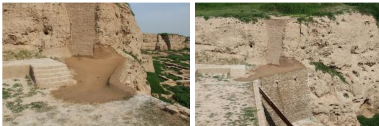
Figure ۴۷. Restoration of water-washed edges of large trench of Shahi City (Fifteenth City)
