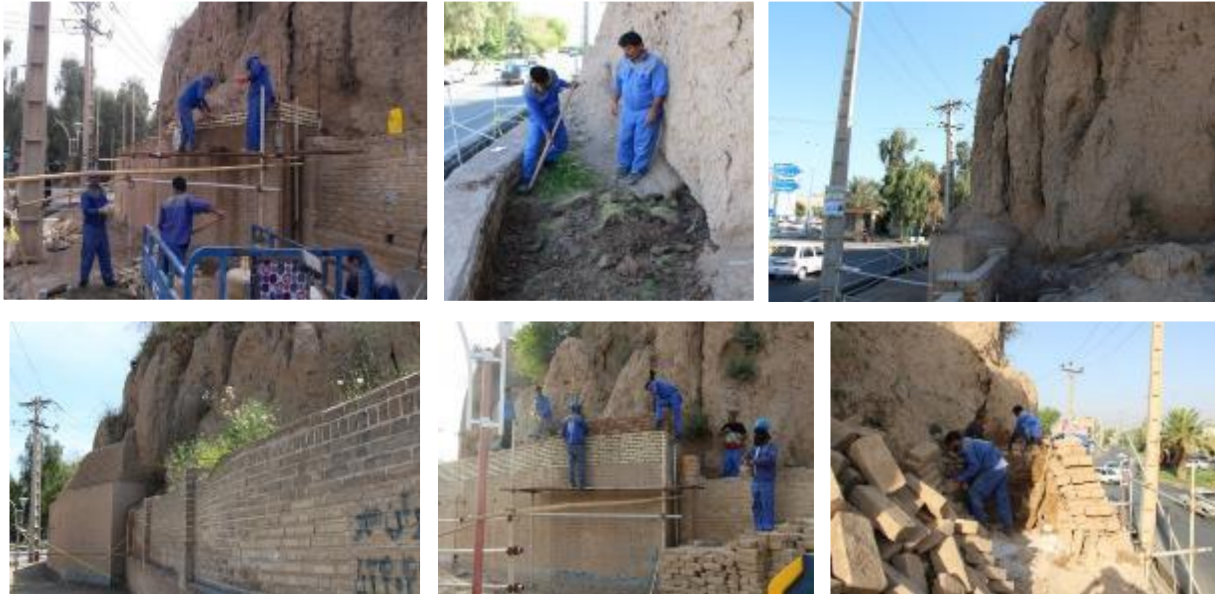
Figure ۵۱ . Protective-restoration Measures on the northwestern tower of Apadana Royal Palace
