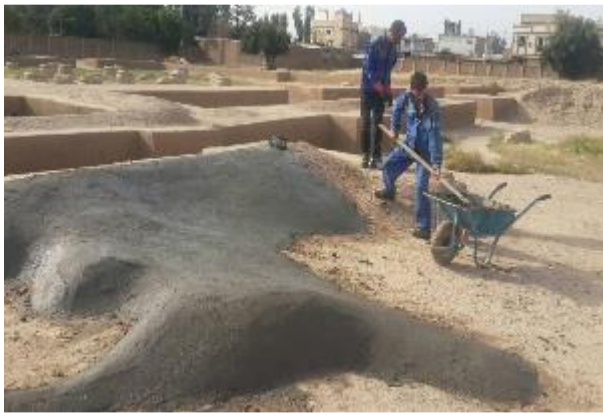
Figure 44. Mud-straw coating of architectural remains of Shavoor Palace
