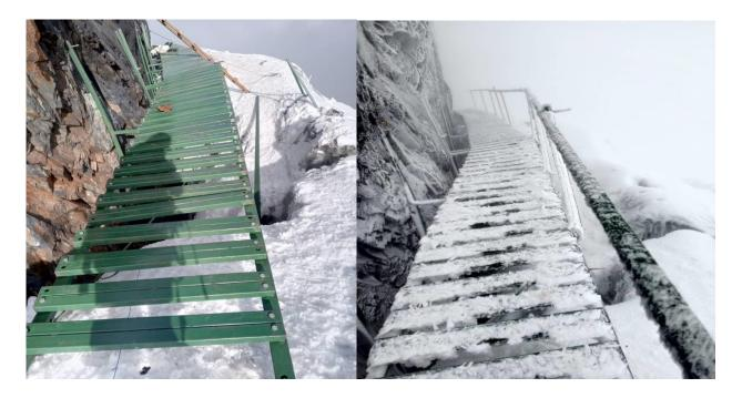
Plate 15: Showing a bridge constructed above Marherita crevasses in RMNP
